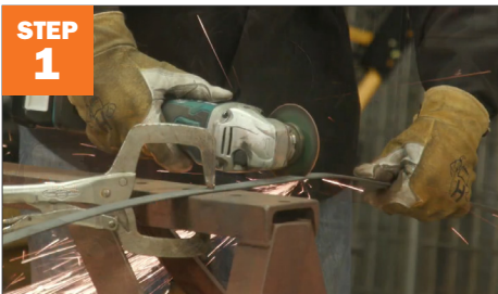
STEP 1 Cut flat bar to desired length.
