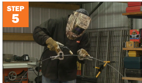
STEP 5 Weld the first ring.
